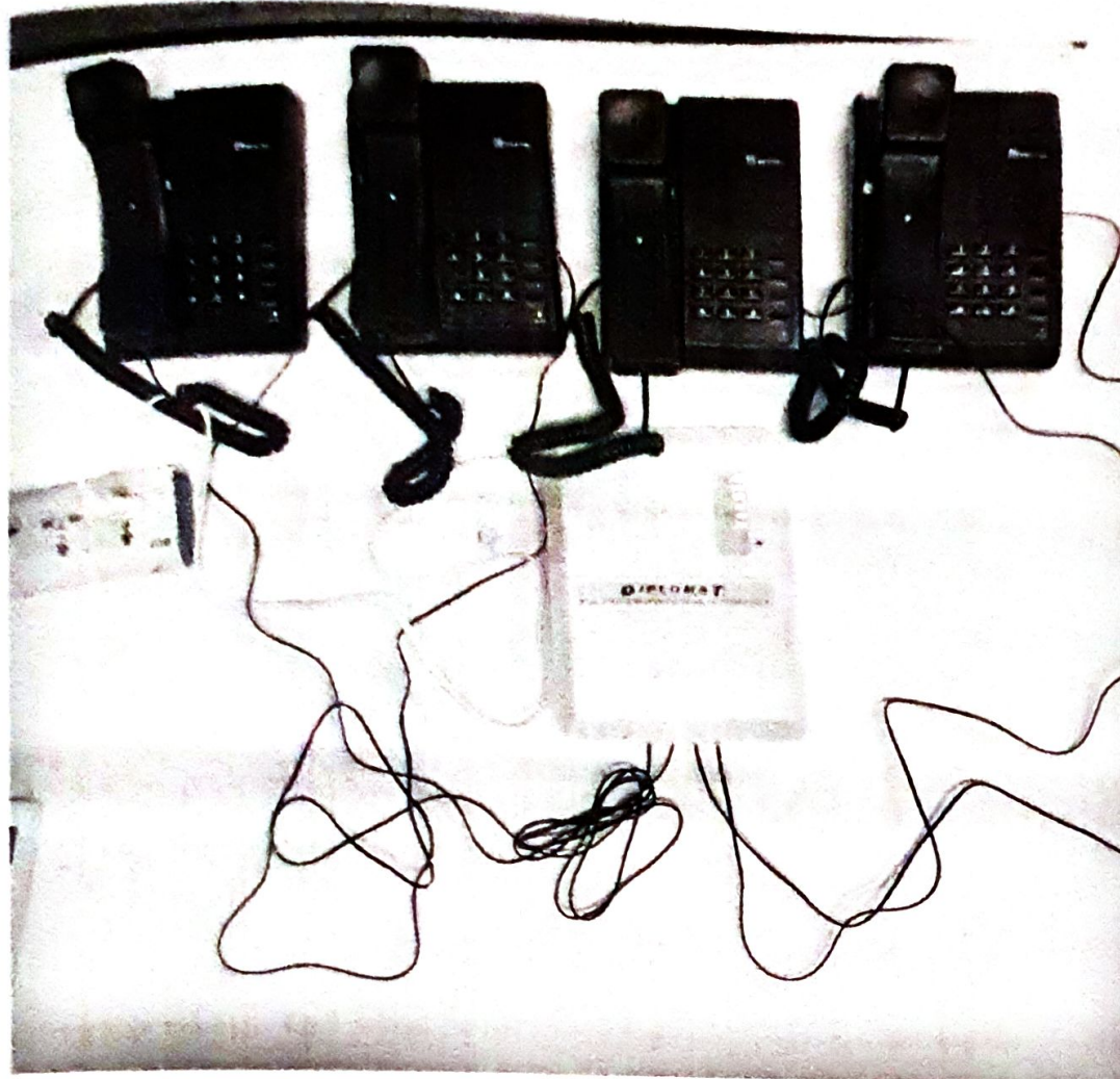
Fig 6.1 Wired Intercom setup
